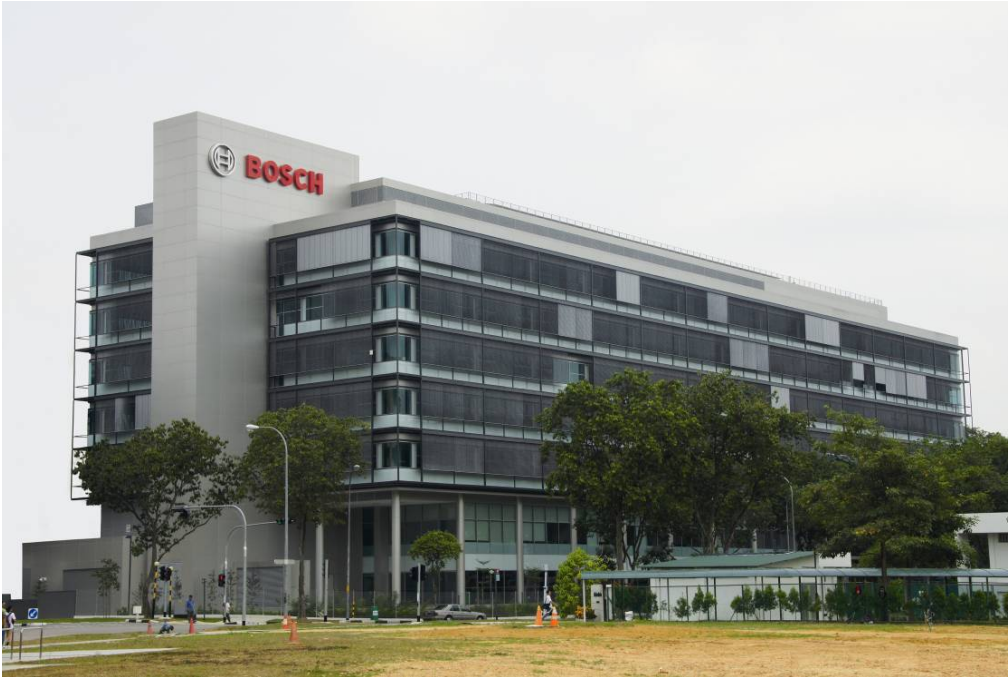
Bosch Southeast Asia regional headquarters – Winner of the Building & Construction Authority Green Mark Platinum Award in 2009, Economic Development Board Solar Pioneer Award in 2009 and 2 nd runner up in the ASEAN Energy Awards 2011
